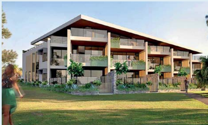
Nine luxury, beachfront apartments are under construction in Lawson Street, Byron Bay.
