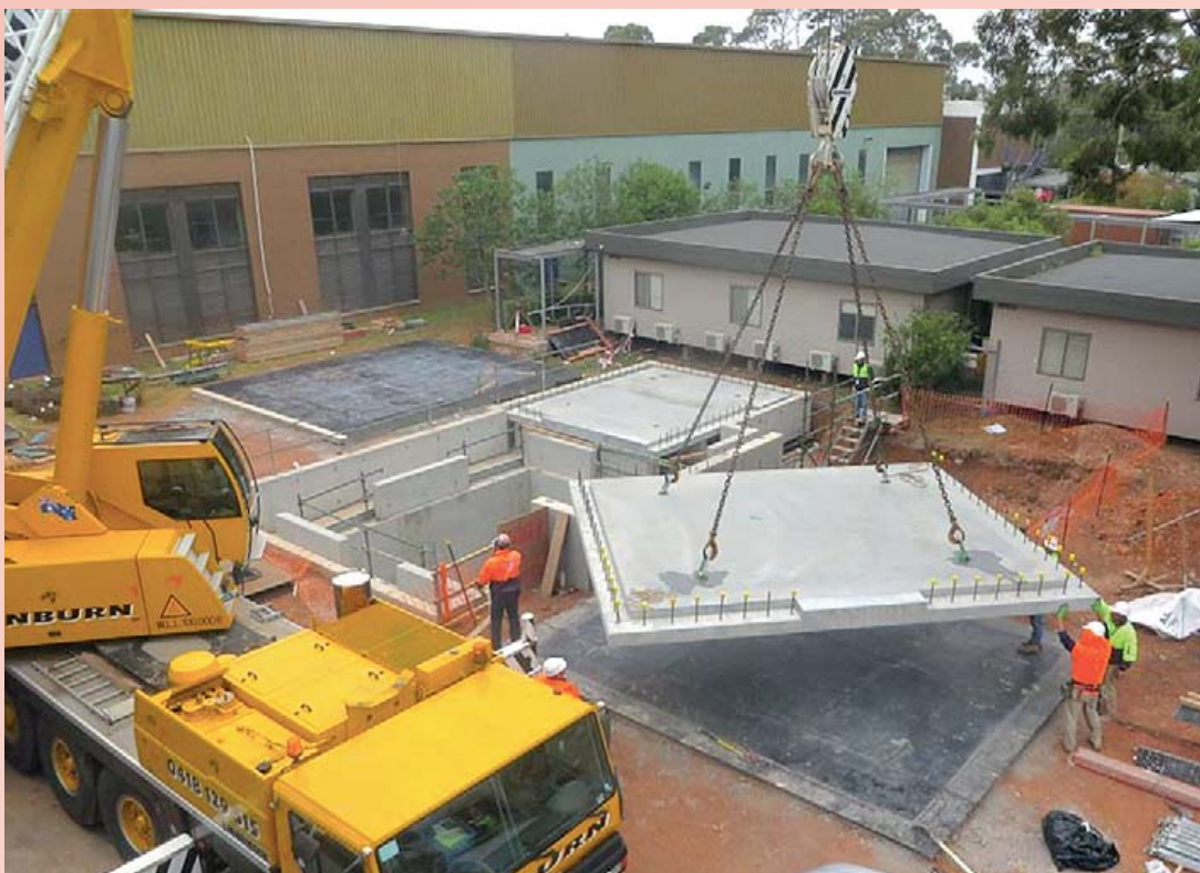
Reverberation chamber under construction for the CSIRO.
